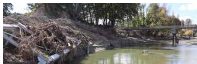
Rissington - old temporary bridge foreground, new temporary bridge background
